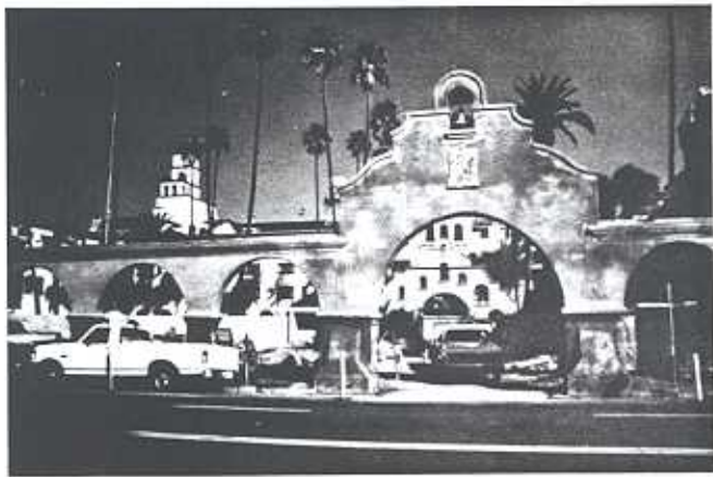
New Structures Should Relate to Historic Riverside.
