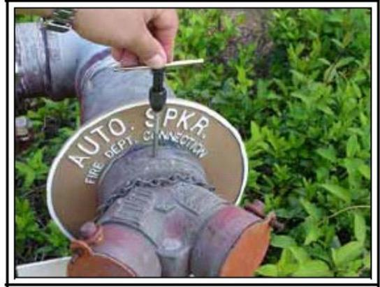
11. Measures the total thickness through the case and pipe thread so that a stainless-steel tamper resistant bolt can be inserted, not to exceed 1/2 inch into the water flow of the pipe. A tamper resistant bolt is designed to be tightened with a flat head screwdriver but cannot be loosened.
