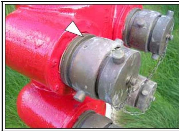
3. Remove the set screw. Please note that this is a very small item shaped like a hockey puck. A pan or tray placed under the connection may capture any small parts from falling onto the ground.
