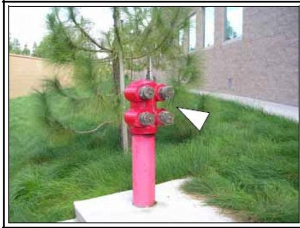
2. Turn the FDC connections so that the Set screw faces upward
