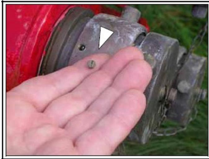
7. Apply a small amount of thread locking chemical on the thread of the set screw per manufacturer directions. Red thread locker is the strongest product.
