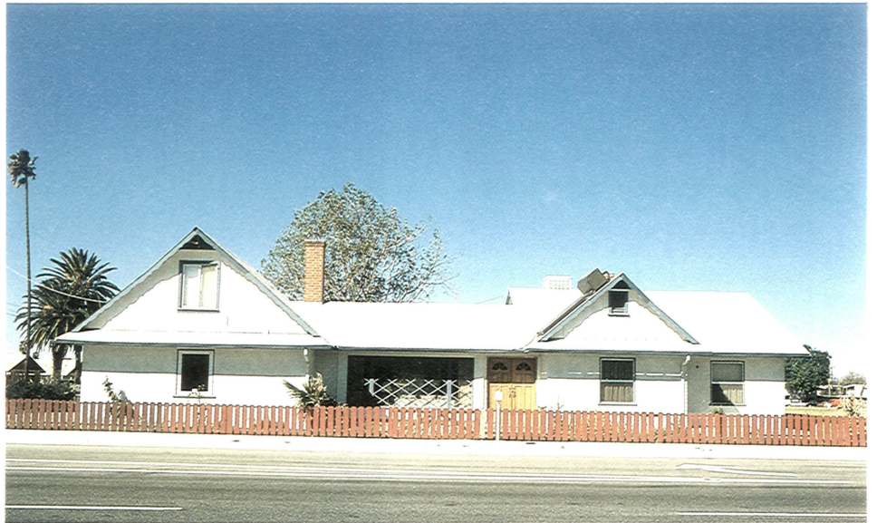
Riverside Energy Demonstration Center
