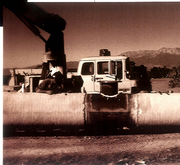
Dufferin Avenue water transmission line construction.
